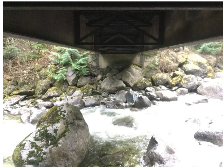
Right Bank Abutment when facing downstream
