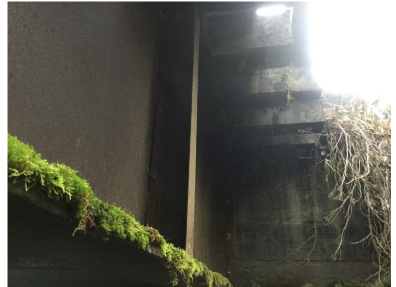
Stiffener located 1880mm from girder end on right bank and 1940mm on left bank
