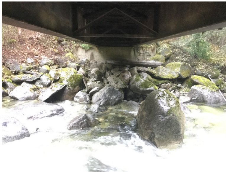
Left Bank Abutment when facing downstream
